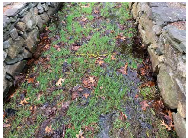
4 Brickyard Circle - 2 (Drainage Course)
