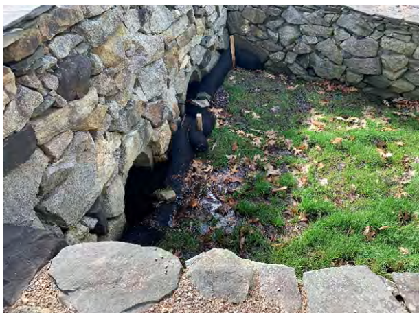
4 Brickyard Circle - 1 (Drainage Course)
