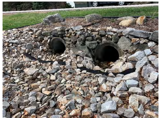
64 Gundalow - 2 (Drainage Course)
