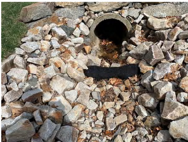
64 Gundalow - 1 (Drainage Course)
