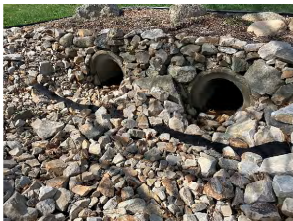
64 Gundalow - 2 (Drainage Course)
