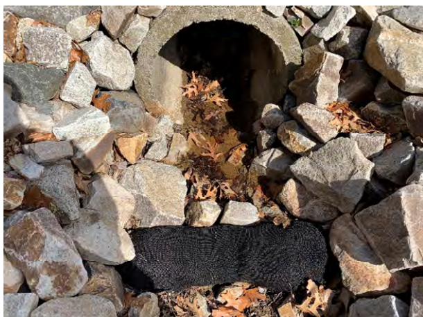
64 Gundalow - 1 (Drainage Course)
