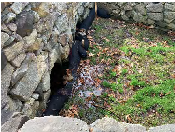
4 Brickyard Circle - 1 (Drainage Course)
