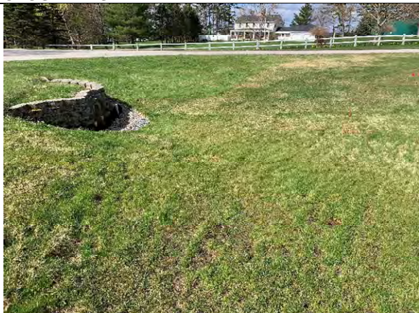
29 Gundalow - 1 (Drainage Area)
