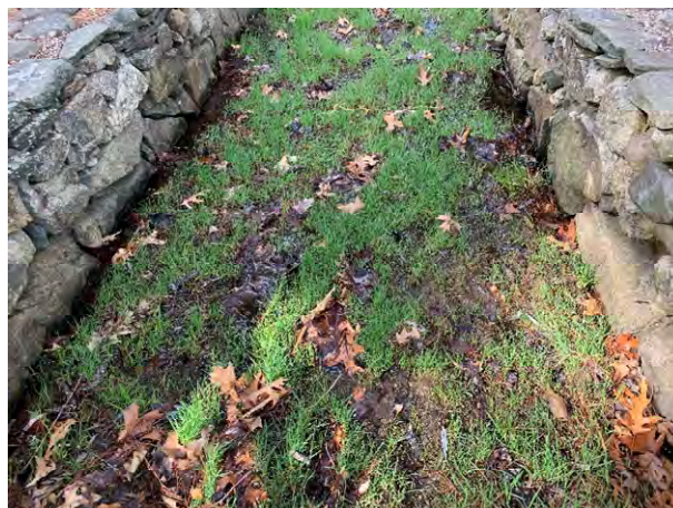
4 Brickyard Circle - 2 (Drainage Course)
