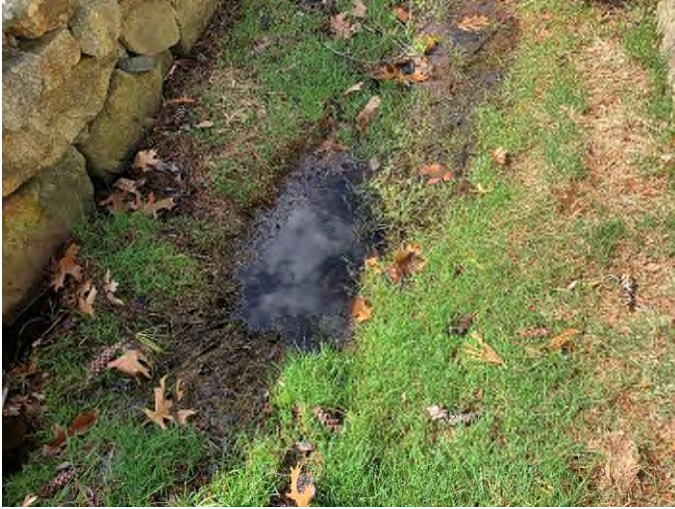
4 Brickyard Circle – 3 (Drainage Course)
