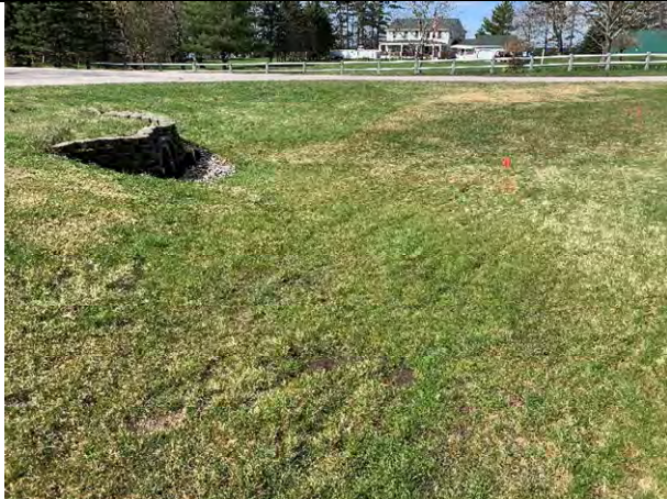
29 Gundalow - 1 (Drainage Area)
