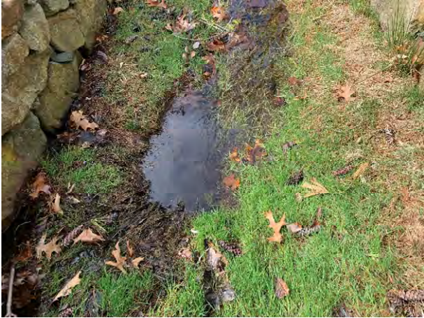
4 Brickyard Circle – 3 (Drainage Course)
